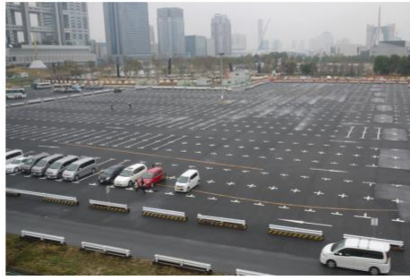
Guard access to parking
